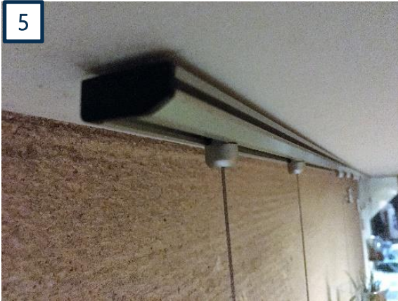
Attach a cap to the end of the rail to prevent the wire from falling off. * The photo shows the display wire
